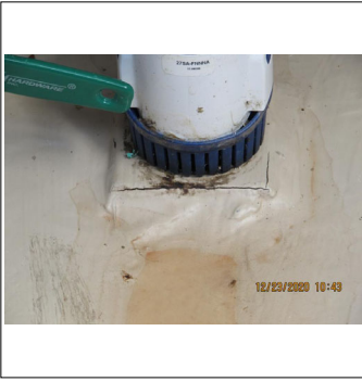
Cracked Fairing Puddy for Bilge Pump Mount directly above Stern CL Impact
