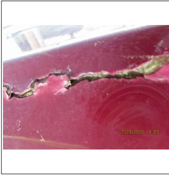
Close up of Inboard Fracture Partial
