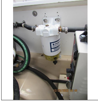
Fuel Filter with Poly sight bowl in Generator space
